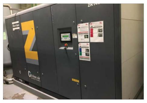
Figure 5: Installing a smaller oil-free rotary screw air compressor, with a heat-of-compression dryer, saved energy in the PET system.
