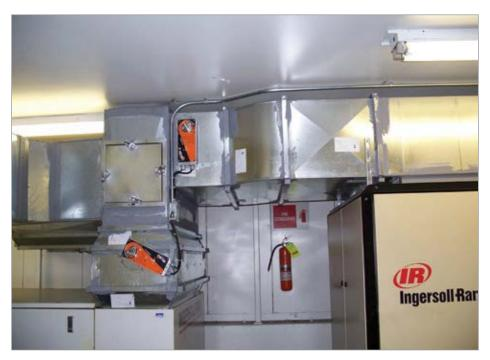
Figure 3: A heat recovery ventilation system saves natural gas costs in winter.
