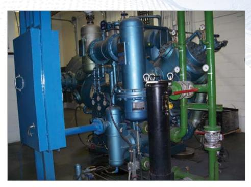
Figure 2: The 600 hp 600 psi PET air compressor consumed significant power.
