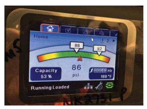
Figure 4: VSD air compressor control increases system efficiency.
