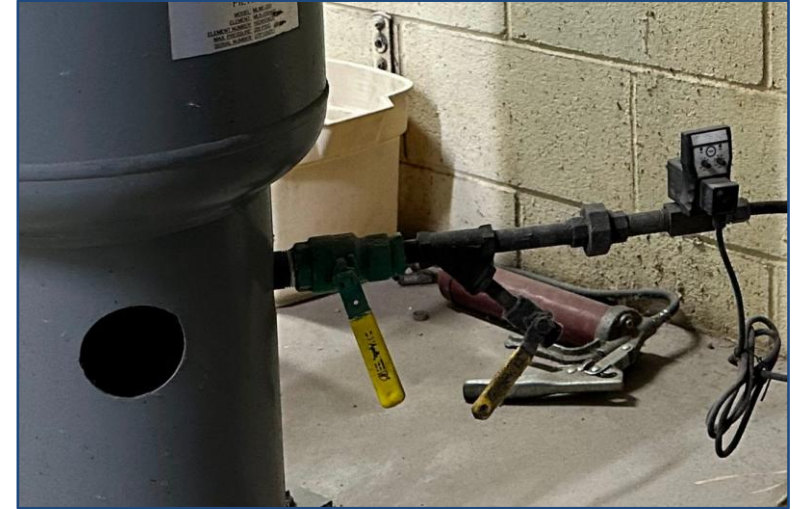
Field finds: a manual valve bypassing the drain to a bucket (top) · a bypass teed around a drain — one cracked valve from a 24/7 leak (bottom)
