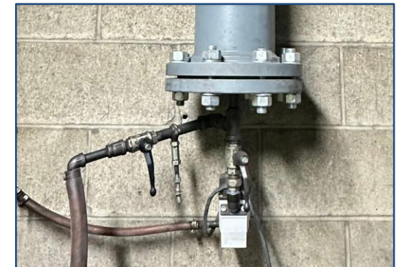
Field finds: a manual valve bypassing the drain to a bucket (top) · a bypass teed around a drain — one cracked valve from a 24/7 leak (bottom)
