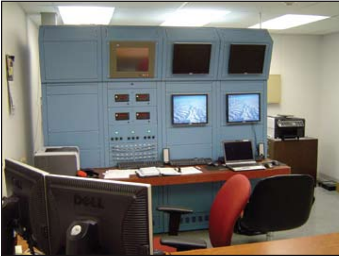
The Command Center Can Simulate All Operating Conditions
