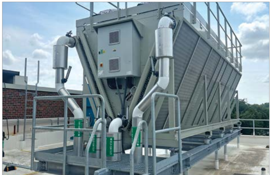
A fluid cooler installation showing piping connections and the control panel
