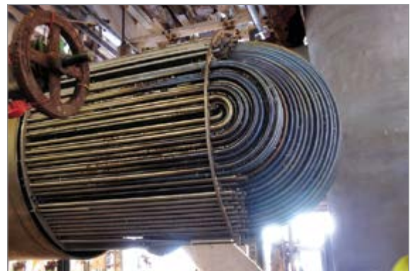
The tube bundle of a heat exchanger
