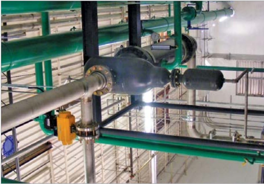
A pipeline-style aftercooler mounted in customer piping (Credit: Alnitak3)
