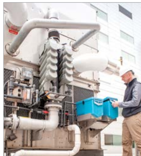
This evaporative, closed-circuit fluid cooler is equipped with a factory-mounted solid water treatment system, designed to improve water management, reduce maintenance requirements and support reliable thermal performance.
