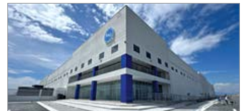
Baltimore Aircoil Company's manufacturing facility in Ciénega de Flores, Nuevo León, Mexico
