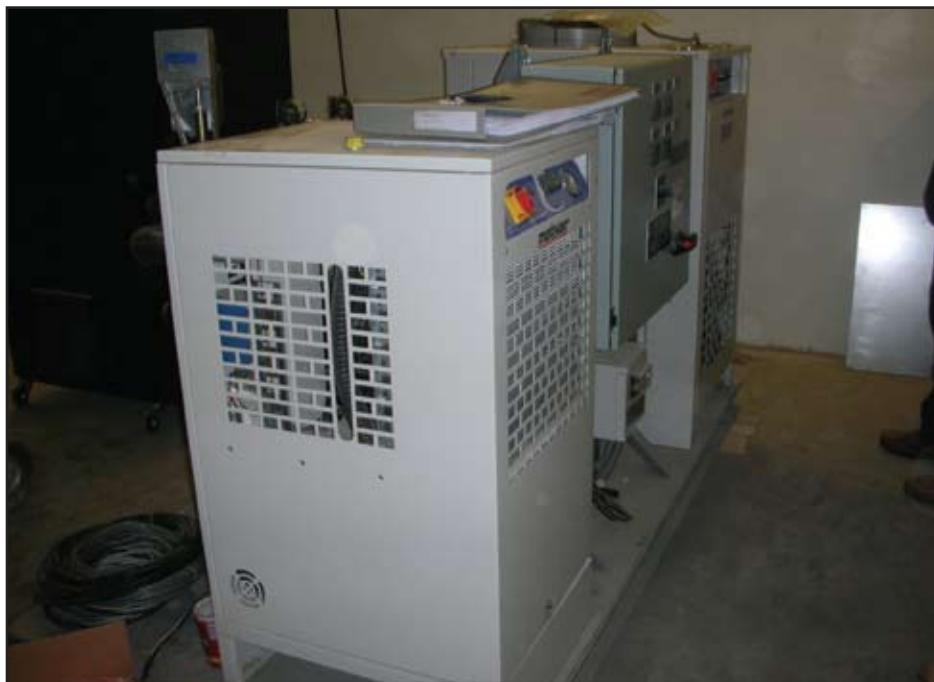
The High-Pressure Dryer, Heater and Cooler Package
