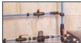
Aluminum air system piping with connections that require no special tools or pipe threading. Courtesy Transair
