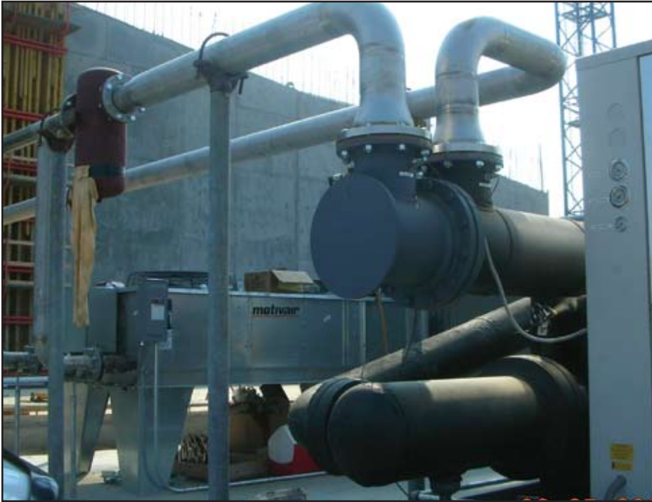
The Air-cooled Aftercooler and Cycling Refrigerated Dryer Ensure Dry Air
