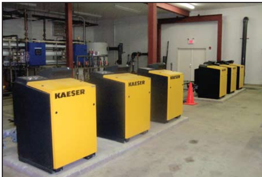
Applied Water Management's System Uses Six Kaeser Com-paK Plus Tri-lobe Blowers
