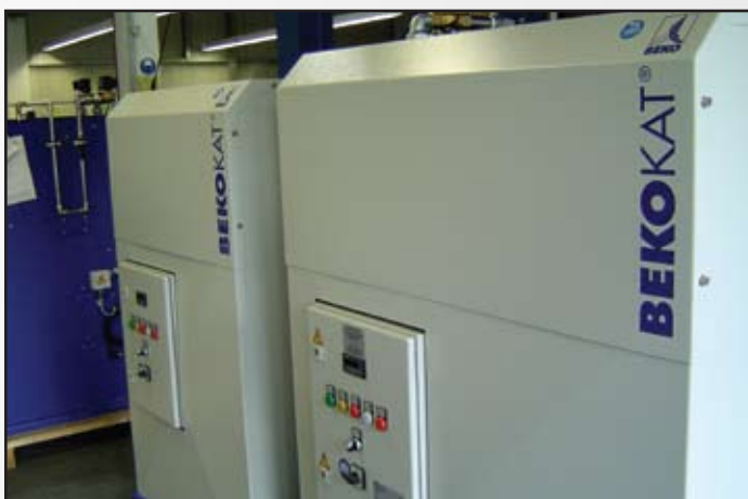
The BEKOKAT uses a unique design, with a catalytic converter, to ensure oil-free air to 0.003 mg/m3
