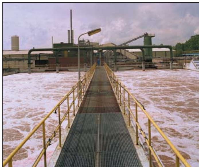
Wastewater Treatment Plant Aeration
