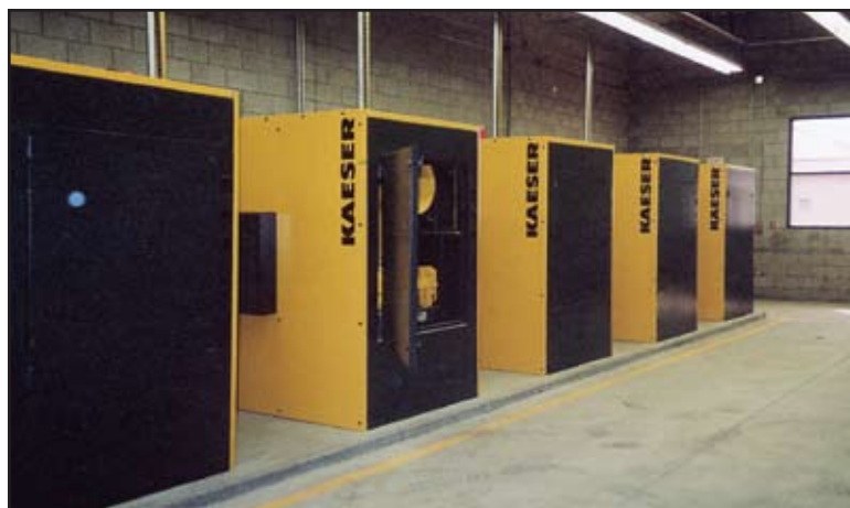
Palm Valley WRF has an installation of six Kaeser 100 hp Omega-pakS Blowers
