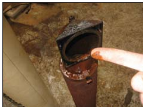
Poor maintenance led to blocked air filters and dryers creating a pressure drop of 35 psig
