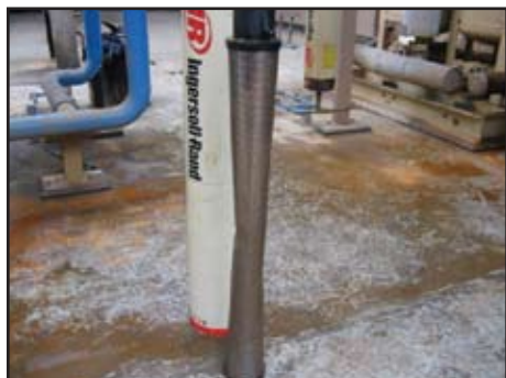
A damaged filter element
