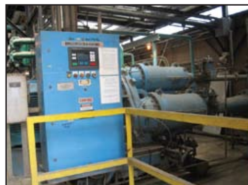
The turn-down controls made this centrifugal oil-free compressor consume 70% of full-load electrical capacity while operating at 40% load — 24 hours per day.
