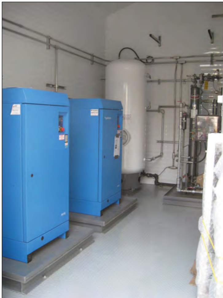
This building contains redundant rotary vane air compressors, a wet air receiver and a regenerative desiccant dryer — all under a PLC controller for remote control.
