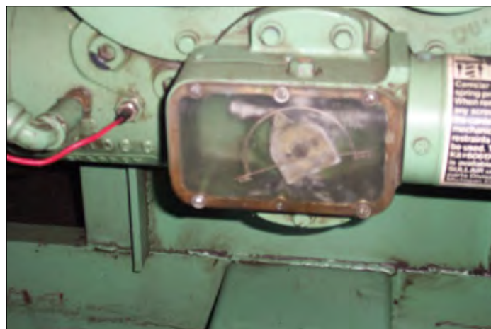
Capacity Controls like this are controlled by a simple screwdriver adjustment. Incorrect adjustment can greatly affect the efficiency of the compressor.
