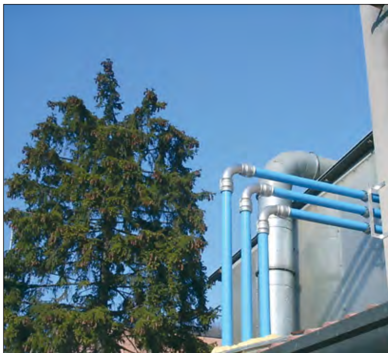
Installed Aluminum Piping.
