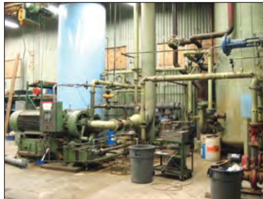
The 700-hp centrifugal compressor used to be operated almost 24 hours a day but by early 2007 was only used once or twice a week.
