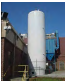
Air receiver tank upgrade.
