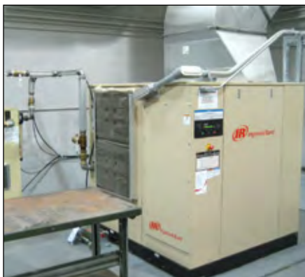
The new system included a 100-hp, fixed-speed rotary screw compressor and a cycling refrigerant air dryer.
