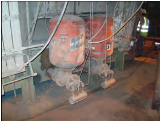
Piston Return Reservoirs installed on BIG BLASTER® XHV TORNADO Air Cannons.
