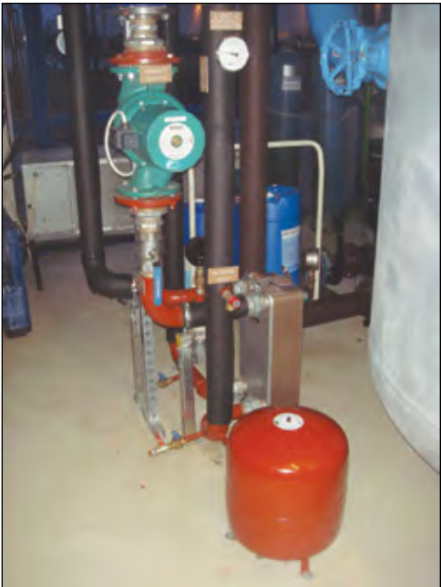
Free-cooling Plate-and-Frame Heat Exchanger
