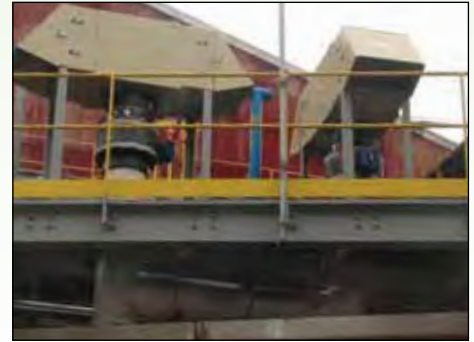
Ingersoll Rand Centac® Dual Inlet Filter Assemblies
