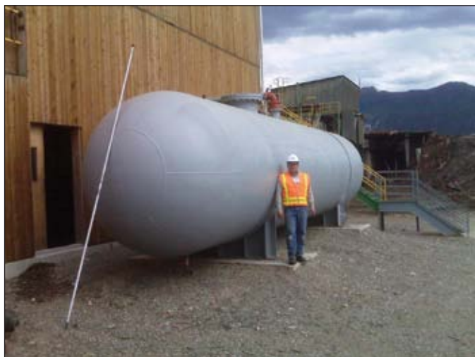
Dusty Smith, P.E., (Director of Engineering at Pneu-Logic), stands in front of an air receiver installed to help deliver large volumes of compressed air instantly to meet sudden process demands.
