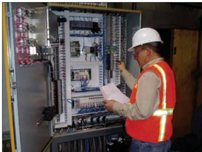
The Pneu-Logic PL-4000 Compressor Sequencing Control System, being programmed by Eric Bessey, P.E. (Chief Project Engineer at Pneu-Logic), manages data from over 40 sensors in each compressor room at Tembec.
