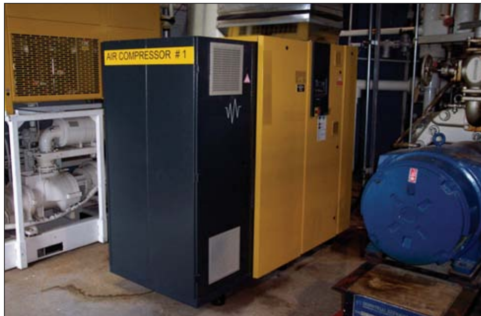
Picture of Milk Plant VSD Air Compressor
