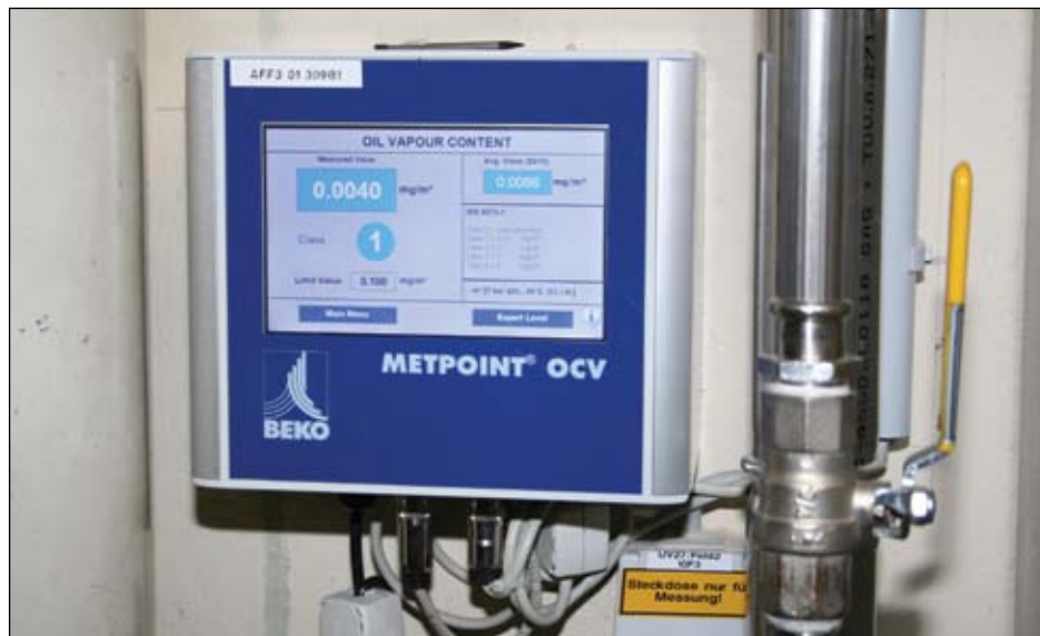
The METPOINT® OCV System installed in a pharmaceutical plant.
