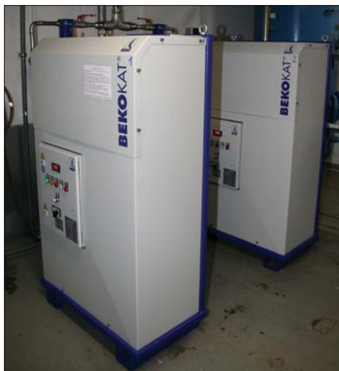
The BEKOKAT® system uses a catalytic converter to ensure hydrocarbon removal.
