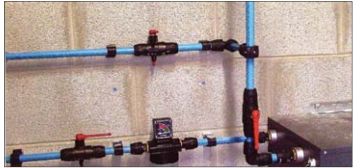
Aluminum air system piping with connections that require no special tools or pipe threading. — Courtesy Transair
