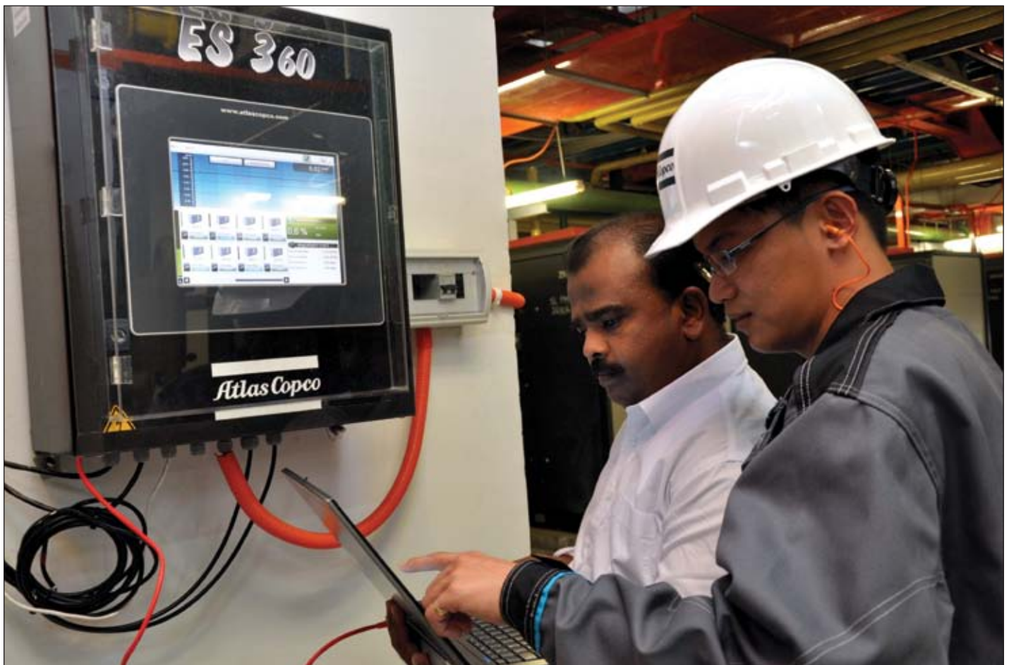
An Atlas Copco System Assessment at a Public Utility Reduced Pressure From 100 to 84 psi.
