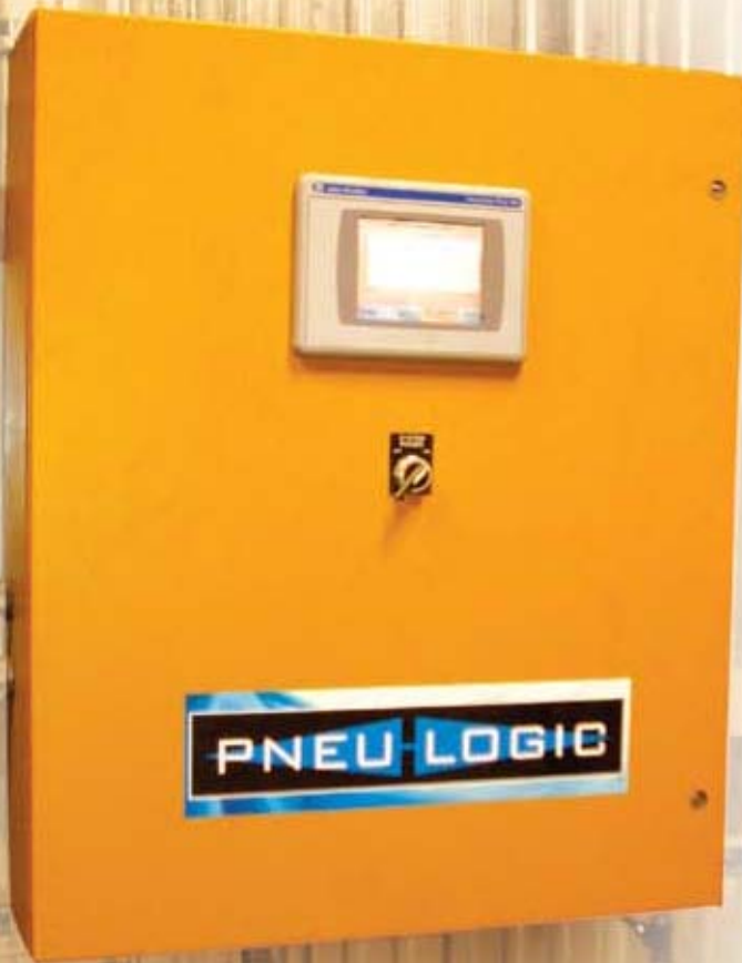
The Pneu-Logic PL1000 Flexible Sequencer Controls up to Eight Compressors.
