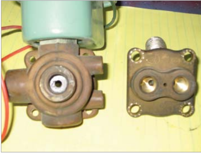
Image 9: A Common 1/4" Solenoid Valve With Small Flow Ports.
