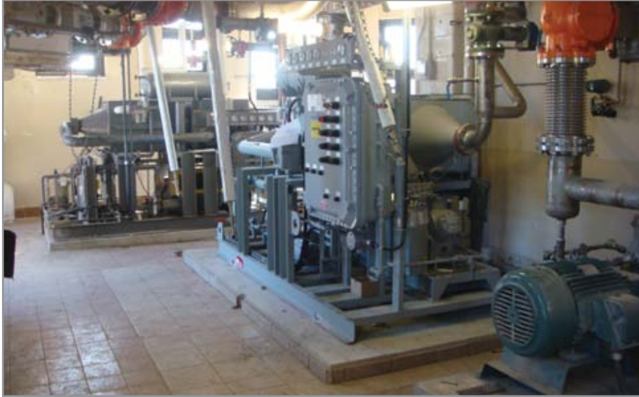
These are PAC-1.7 LDS/40 model dryers installed at the city landfill in Barrie, Ontario.
