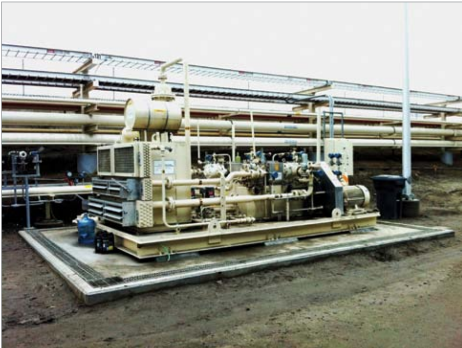
Two-Stage Fuller Vane Compressor as a Vapor Recovery Unit System.
