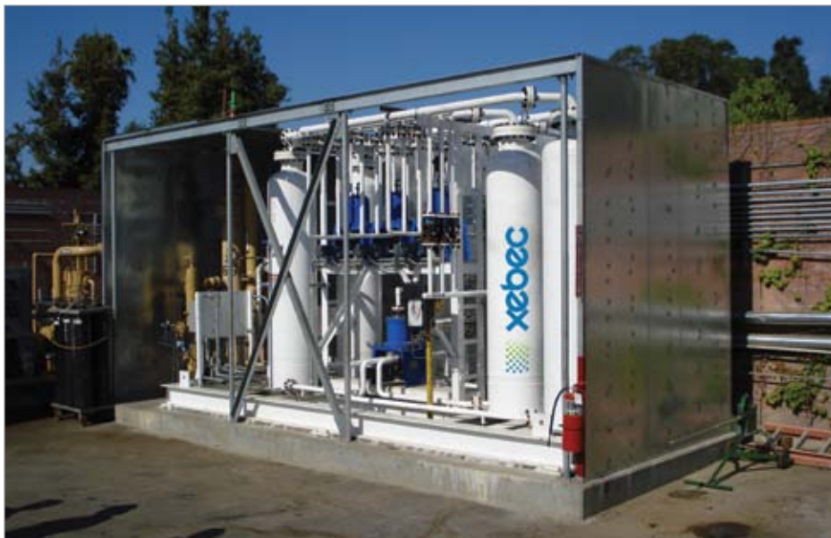
The Xebec compact M-3100 fast-cycle PSA system was the perfect solution to dehydrate field gas at a Southern California oil field.
