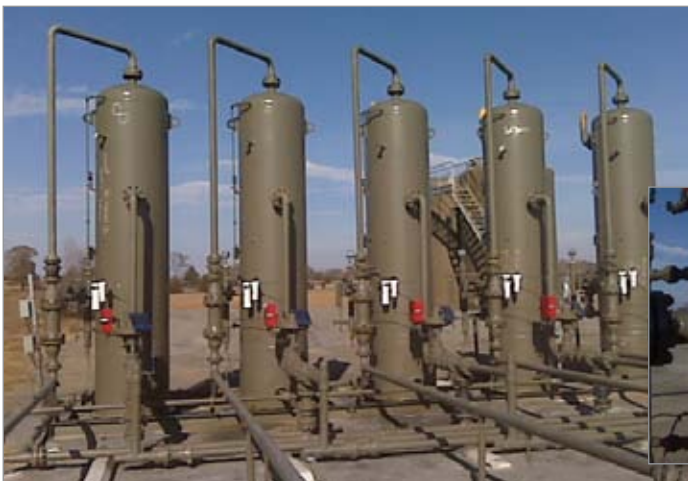
Instrument gas dryers, with 1 Micron Particulate Prefilters, protect valves on production separators.
