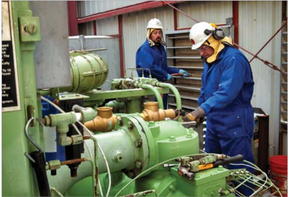
Sullair air compressor start-up and check-out at a food processing plant.
