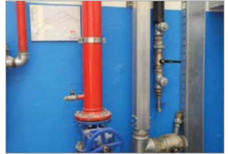
TESEO HBS modular piping for the new compressed air distribution system in the factory of Persico Spa.
