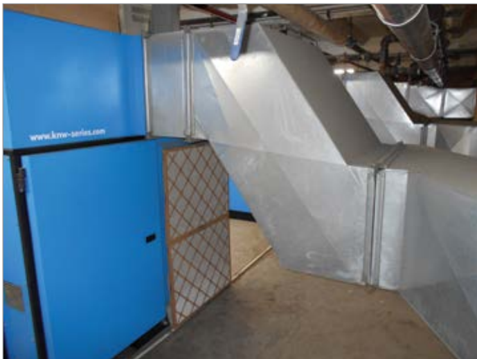
The custom designed rear discharge on each Komatsu KNW series compressors (left) and custom insulated wall plenum (right) directing air into the plant during winter months and to the outdoors during summer months.
