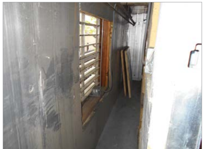
The custom designed rear discharge on each Komatsu KNW series compressors (left) and custom insulated wall plenum (right) directing air into the plant during winter months and to the outdoors during summer months.
