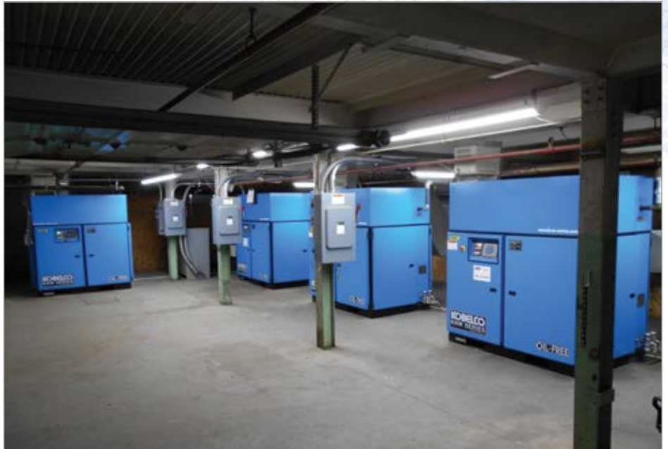
The custom designed Kobelco KNW series oil-free screw compressors provide compressed air year-round, and space heating for 6 months of the year, at International Wire's plating facility.
