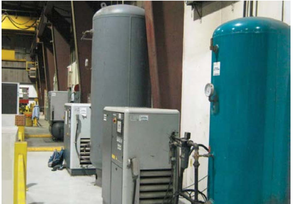
Figure 4: Six smaller air compressors totaling 165 hp were replaced with one 75 hp compressor (and a 75 hp backup).
