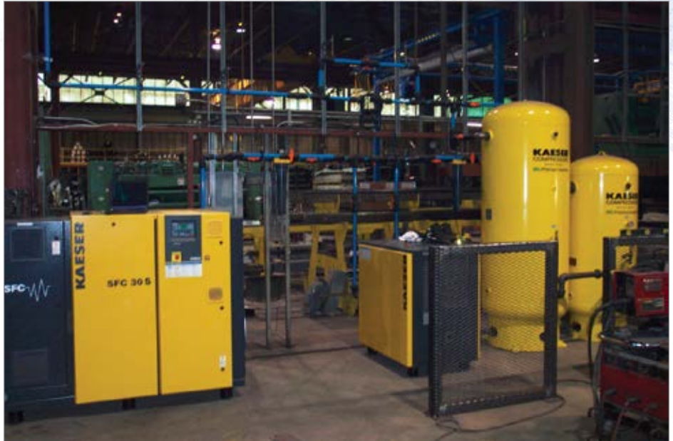
Figure 2: A VSD air compressor, cycling dryer, pressure/flow control valve and storage receivers optimize energy usage.
