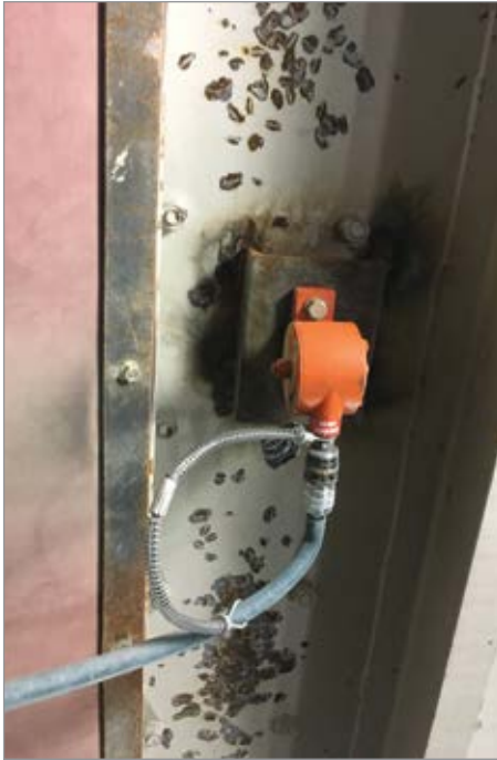
Figure 4: Air vibrators like this could be the reason a second compressor has to run.
