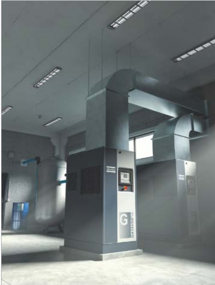
Figure 2: Ducting heat from a pair of compressors
