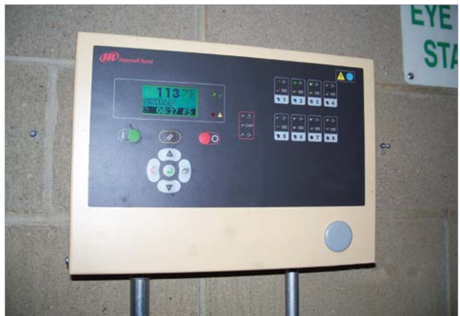
Figure 3: This controller keeps pressure constant while choosing the most efficient compressor.
