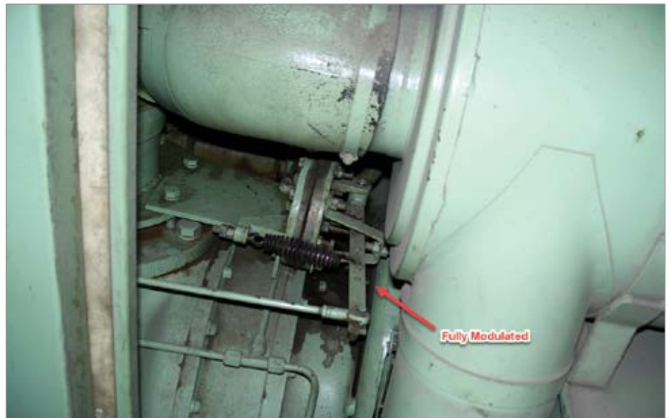
Figure 2: Compressor inlet Fully modulated at poor efficiency.
