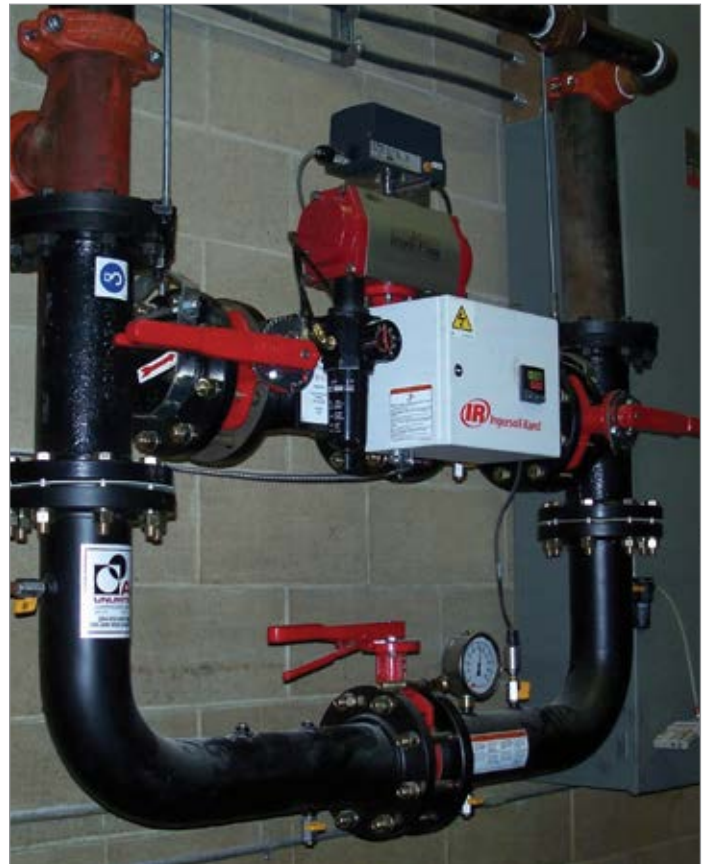
Figure 6: Flow controller reduces artificial demand.
