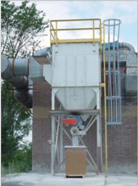
The LST System is a typical pulse jet dust collector for waste product.
