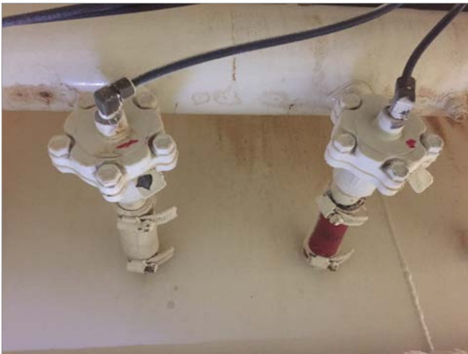
A 20 year-old dust collector with original pulse valve diaphragms. Notice diaphragm tab is painted same color at unit.
