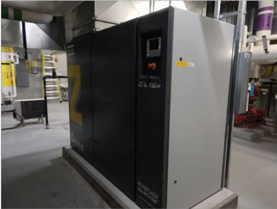
Figure 5: A compressed air dryer is installed internal to the air compressor package, saving floor space.
