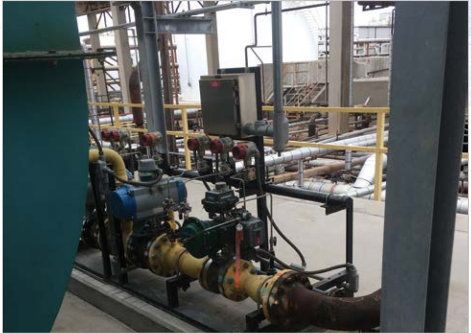
A compressed air leak detection survey can take as many 12 weeks to complete. Engineering tape wrapped around leaks, such as the one shown here, makes them easy to spot for repair.
