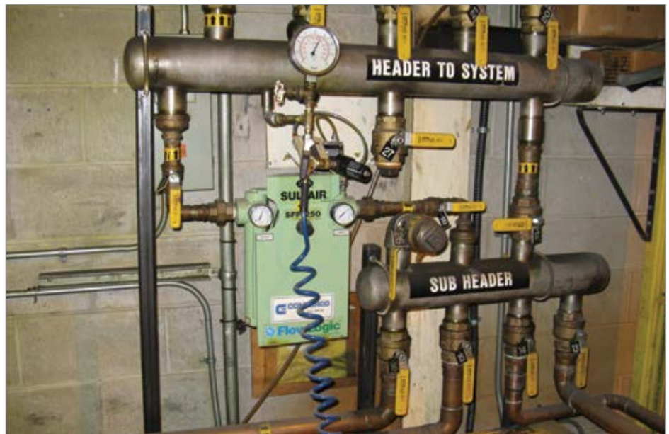
A pressure/flow controller kept plant pressure at a low level and reduced artificial demand.
