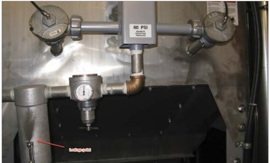
A poorly adjusted blast valve and leakage created problems with this dust collector.
