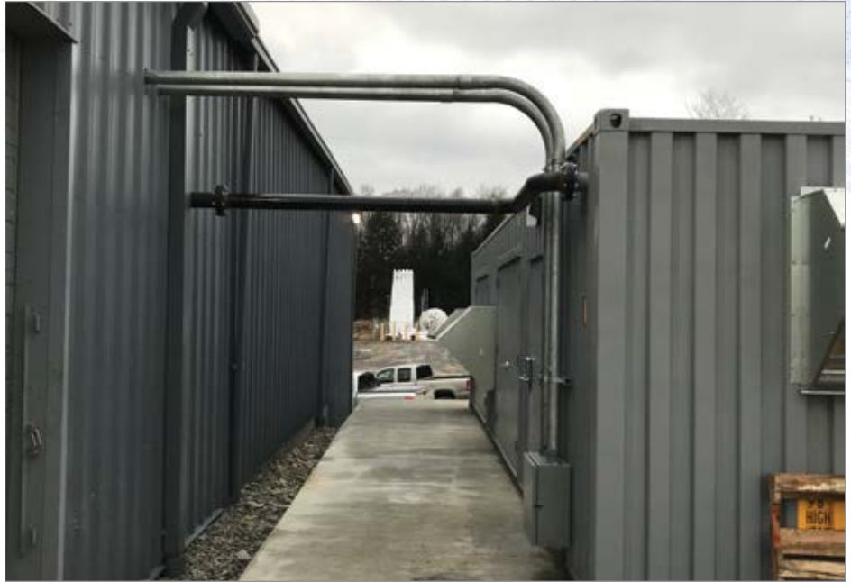
The 40-by-8-foot sea container at GKN houses a complete compressed air system. The unit is located six feet away from the exterior wall of the manufacturing facility.
