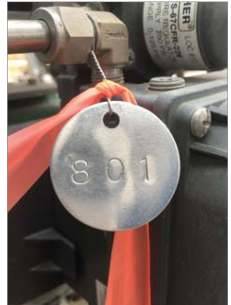
A metal tag with a stamped number identifies the source of a compressed air leak.
