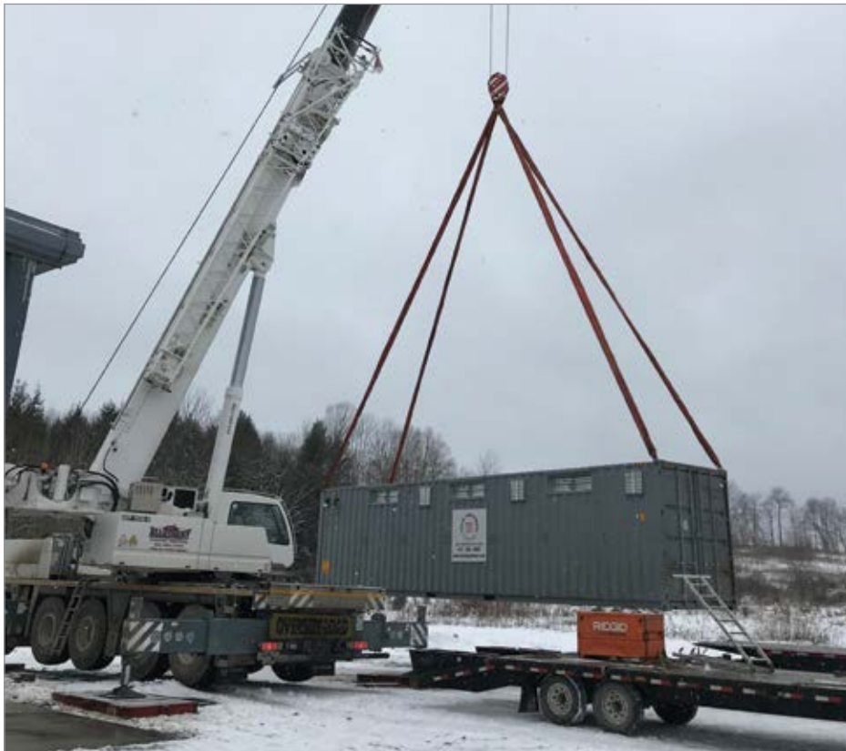
A crane deftly places the sea container into place at GKN. The container houses the entire compressed air system used to meet the air demands of the manufacturing facility.
