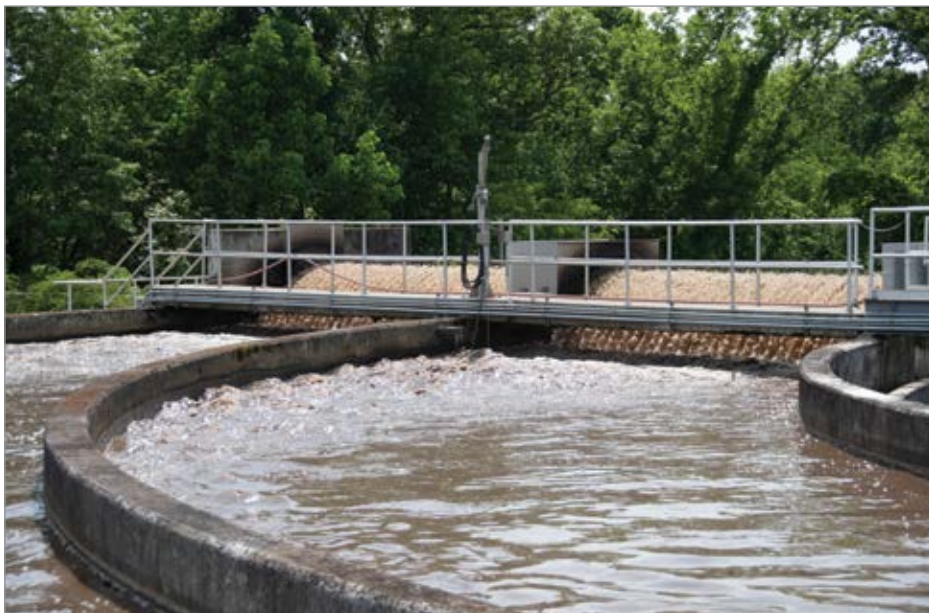
Fayetteville WWTP's split-level oxidation ditches use VFD-controlled surface aerators to save energy and ensure proper aeration.
