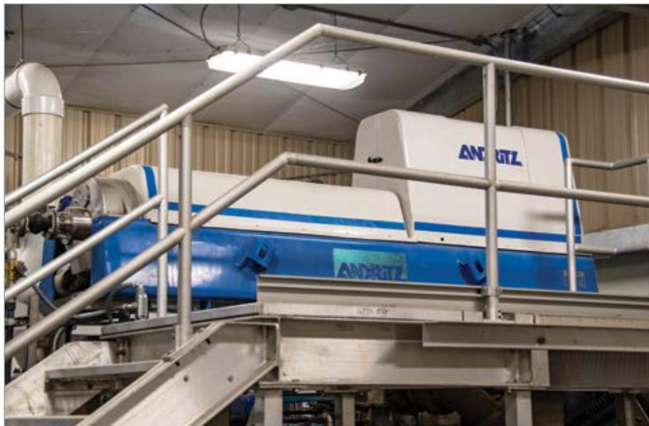
Shown is the high-speed centrifuge used in the dewatering process at the Fayetteville WWTP.
