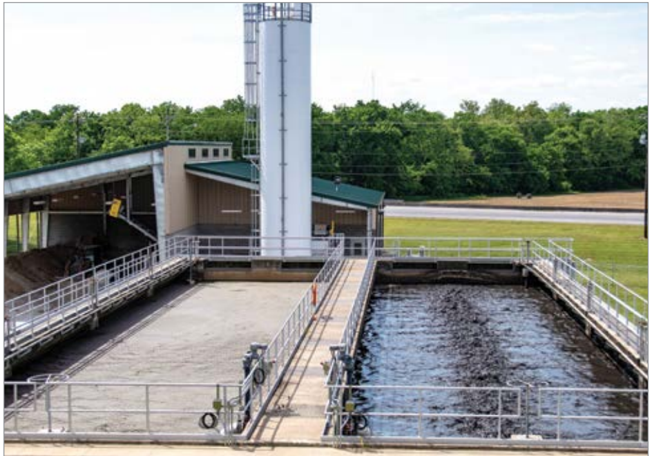
Shown is one of two aerobic digesters used at the Fayetteville WWTP.
