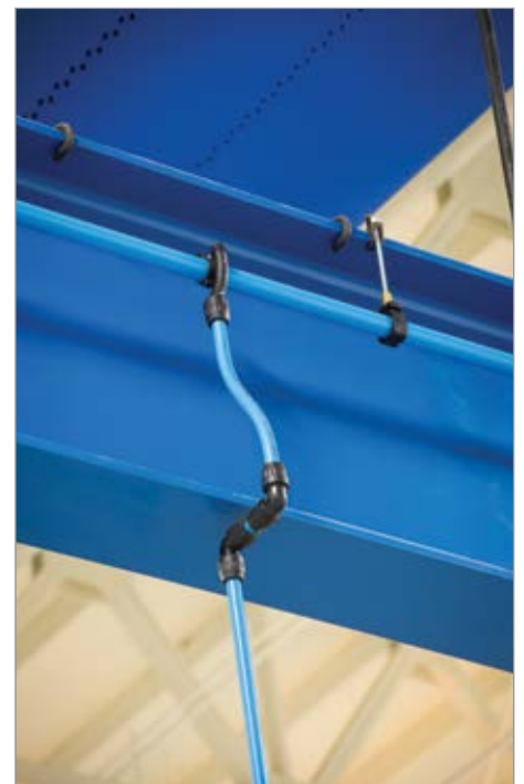
Piping that can be easily bent helps avoid too many elbows in a compressed air system.
