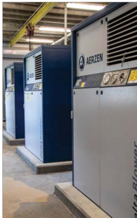
Recently installed aeration blowers play a key role in helping the Fayetteville WWTP optimize its aerobic digesters and achieve energy savings.
