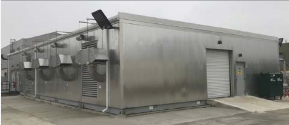
Inlet air hoods protrude from the main modules of the compressed air system at the automotive plant. The overhead door of the modular system provides easy access for maintenance.
