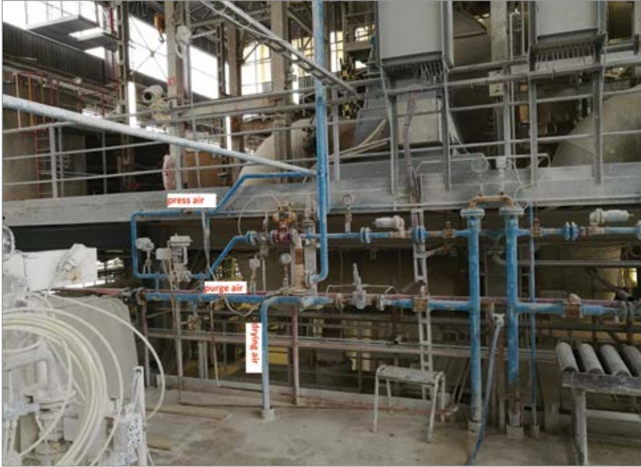
The chemical plant reconfigured its compressed air piping system to allow the newly configured system to deliver air more efficiently and cost effectively at the appropriate pressure to specific press processes.
