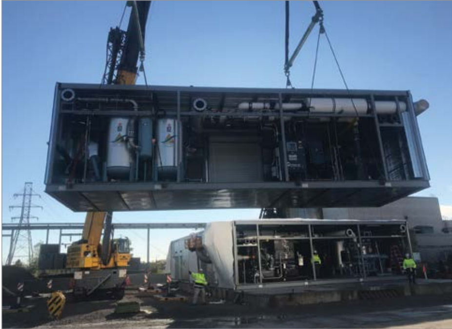
At the automotive plant, modules for the compressed air system are individually offloaded by a crane and set on a foundation.
