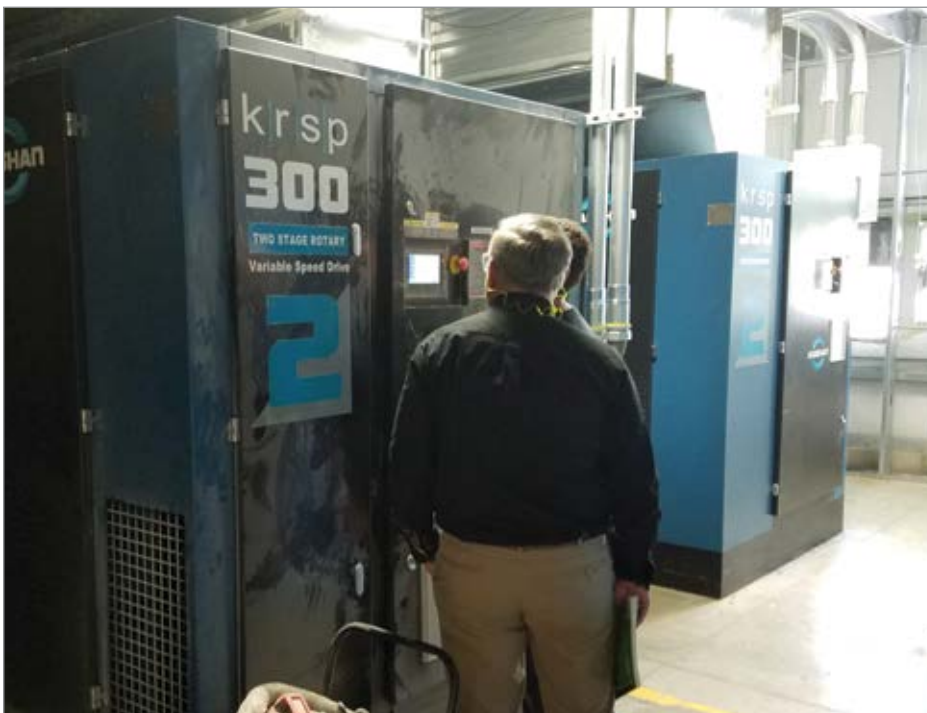
The upgraded compressed air system at AZEK's Ohio plant includes two 300-horsepower VSD rotary screw air compressors.
