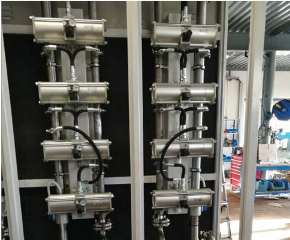
The booster configuration at the chemical plant consists of three rows of four boosters to supply high pressure air to presses used in the process of drying titanium oxide.
