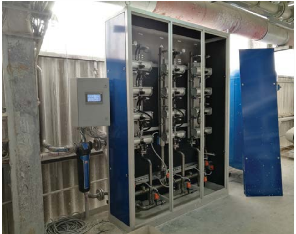
Based on the results of an audit using cloud-based software a large chemical plant replaced a high-pressure system with these pneumatic boosters, allowing it to avoid a costly relocation. The newly configured system is also expected to save the plant $45,000 per year in energy and maintenance costs.
