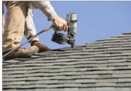
Roofer using an efficient pneumatic nail gun operating from a small gasoline powered or electric powered air compressor.
