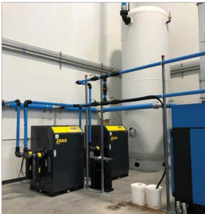
The compressed air system at SCI's Delavan plant includes a 3,800-gallon dry receiver tank. (Photo courtesy of Zorn Compressor & Equipment)
