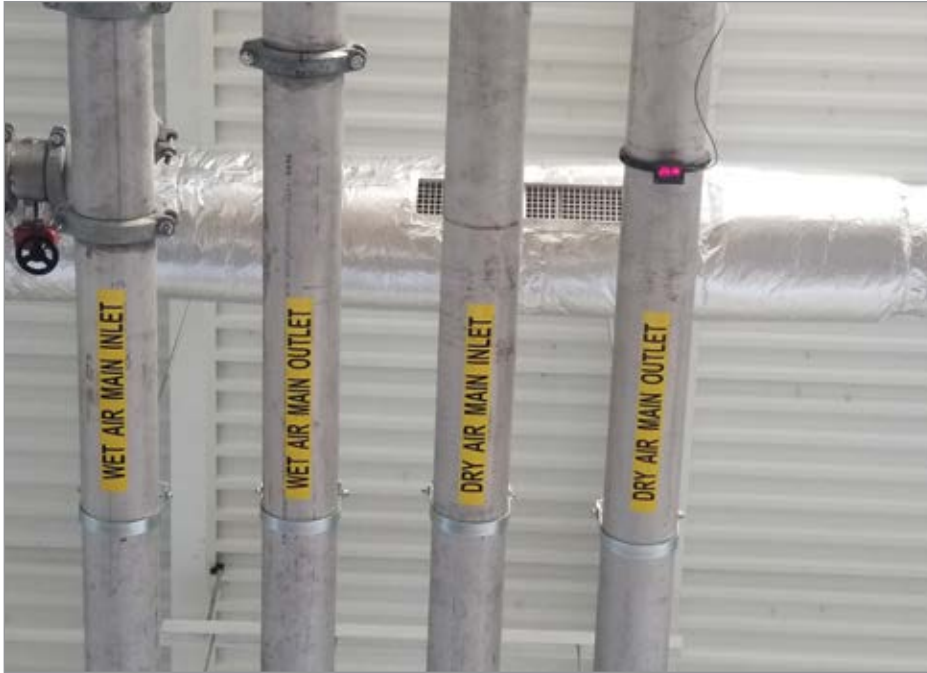
Compressed air flow meter on the main supply header to production.
