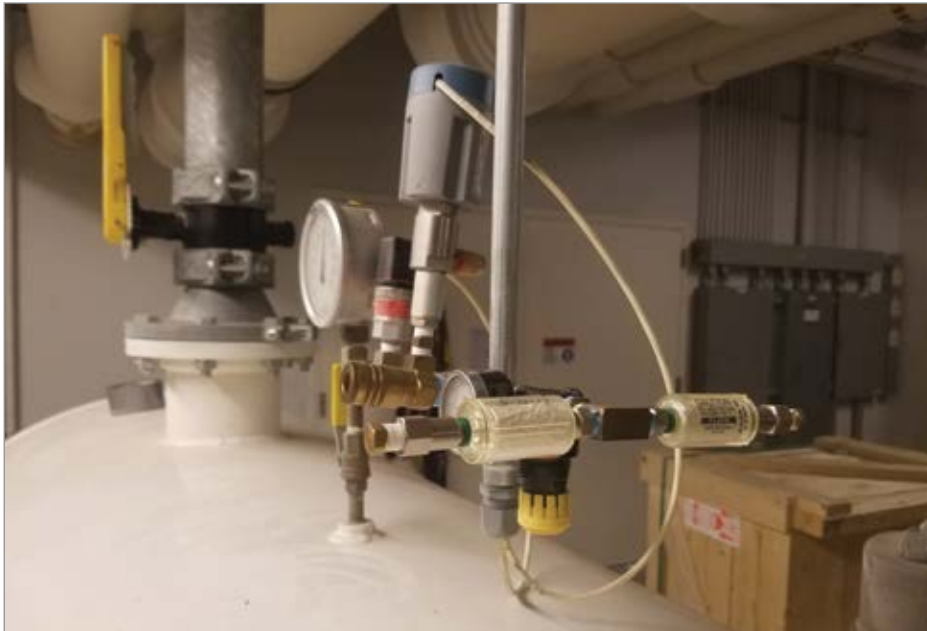
Adding mechanical oil and water indicators on the dry tanks added further assurance of air quality.
