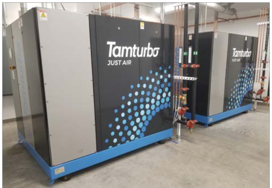
One air compressor as standby/backup. This unit is 100% oil free, with very low maintenance and variable speed drive.
