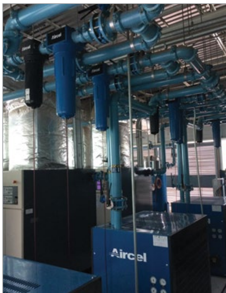
Multiple dryers and an assortment of filters, as well as oil-water separators, address the plant's need for clean, dry air.
