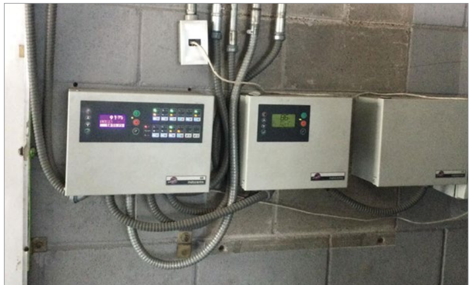
A master controller (left) and a smart controller ensure the compressed air system efficiently delivers air at a stable pressure to plant users.
