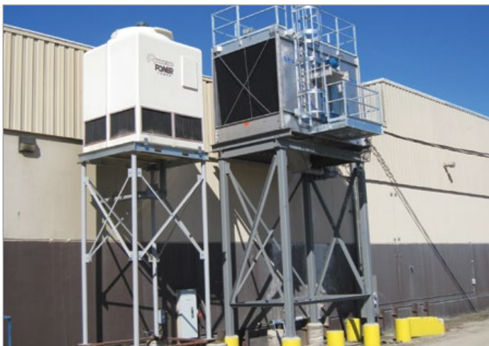
New cooling tower and tower auxiliary equipment.
