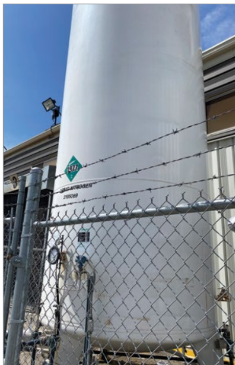
Large Dewar style storage vessels, constructed like a large thermos bottle, have the disadvantage in that a portion of the gas must be vented to atmosphere to control the pressure during periods of plant inactivity.
