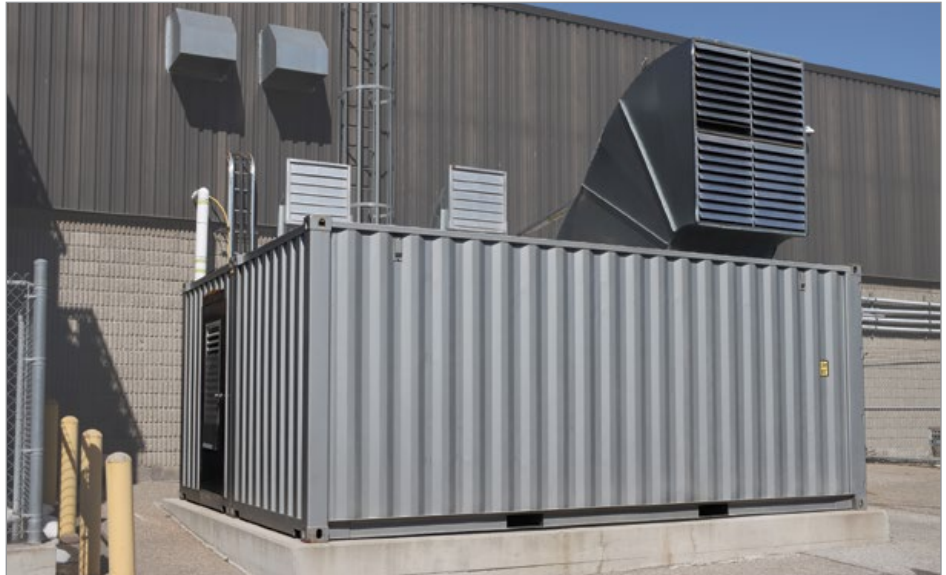
Components of the updated compressed air system at the food processing plant are housed in a BOGE in a BOX container outside the facility.
