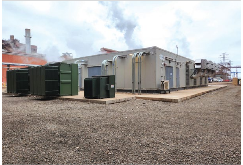
UCA and Envirosep worked together on the final engineering design for the 27,000 scfm compressed air plant.
