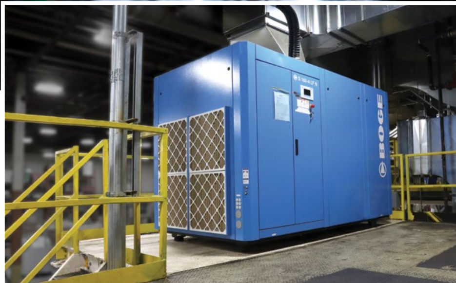
The compressed air audit led to the installation of an energy-saving rotary screw VSD air compressor.
