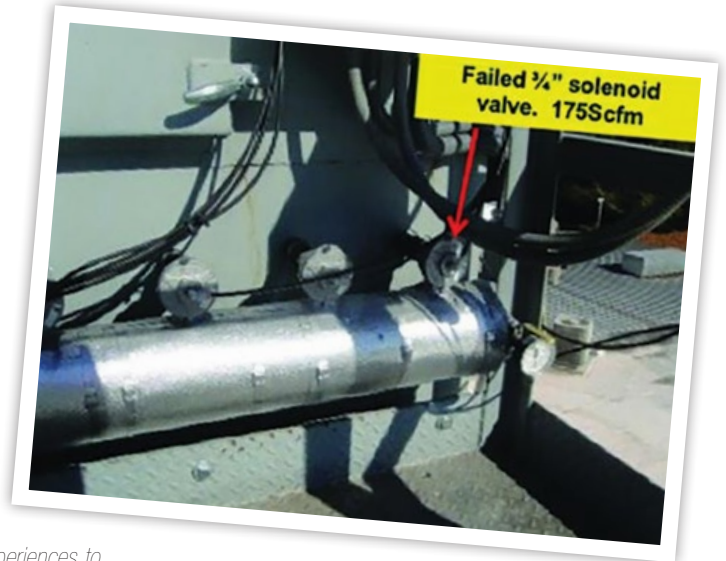
The pilot valve assembly on a 3/4" solenoid valve on the Flour dust collector located on the roof has come disconnected allowing 175 Scfm of air to continuously blow. Photo credit: Mike Lenti, Senior Auditor, Compressed Air Consultants
