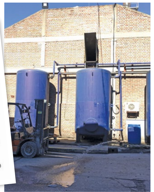
Two thousand liters (500 gallons) of water came pouring out of the compressed air storage tank. Photo credit: Marcelo Cassani, Pneumac Service S.A.
