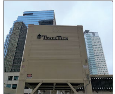
A Tower Tech cooling tower installation.
