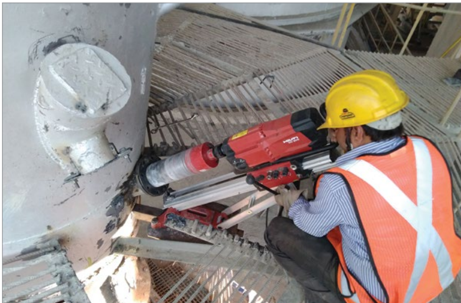
Core drilling during production by a trained technician.
